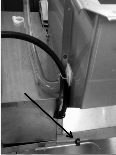
Figure 1 1 Cube Probe Location
